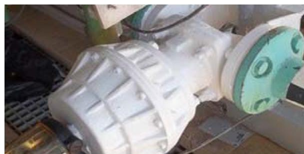
Equipment coated with the high layer coating obtained in the reaction of modified novolac epoxy.
